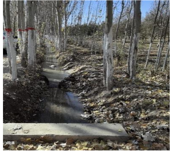
拟建渠道现状
