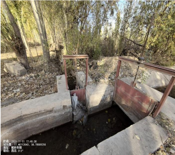
拟建渠道现状
